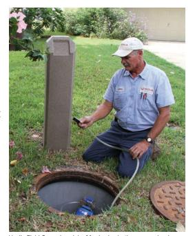
Veolia Field Supervisor John Morris checks the vacuum level in Crystal River's AIRVAC sewer system as part of a scheduled maintenance program.
