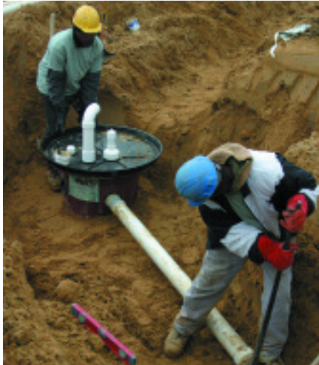
Left: Each valve pit typically serves two connections. Laterals are connected to each home and operate on gravity flow principles. Right: The AIRVAC technology is easily expandable and will include the Bay Creek Marina.
