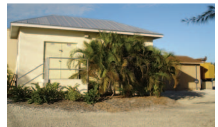
This vacuum building (foreground) on Stock Island, Fla. — the only part of the vacuum sewer system that requires power — houses four pumps, which provide vacuum pressure for the entire collection system. The building is designed to withstand a Category 5 hurricane and is connected to a diesel-powered, 150,000 W/150 kW standby generator (right).
