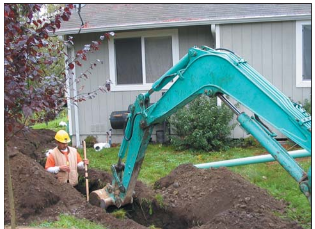
Typical side sewer installation job site.
