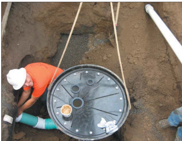
Connecting side sewer to valve pit.
