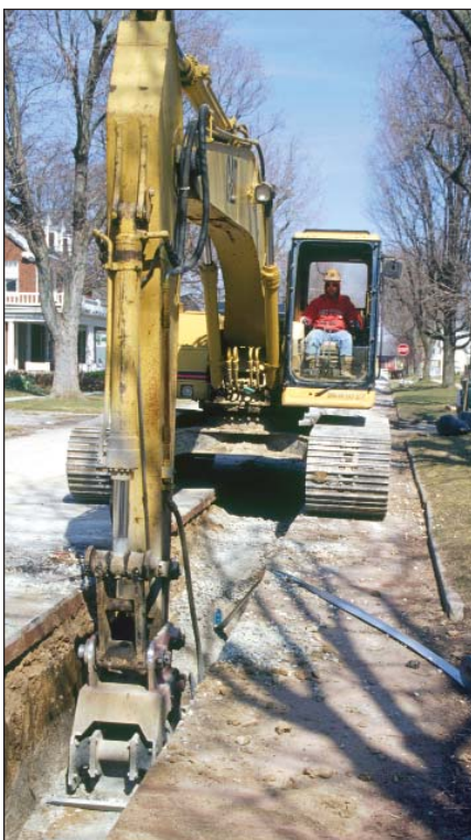
Vacuum sewer lines typically require much shallower depths (4-5 feet) than do gravity-flow sewers. The shallow trenches mean less neighborhood disruption, greater worker safety and lower installation costs.
