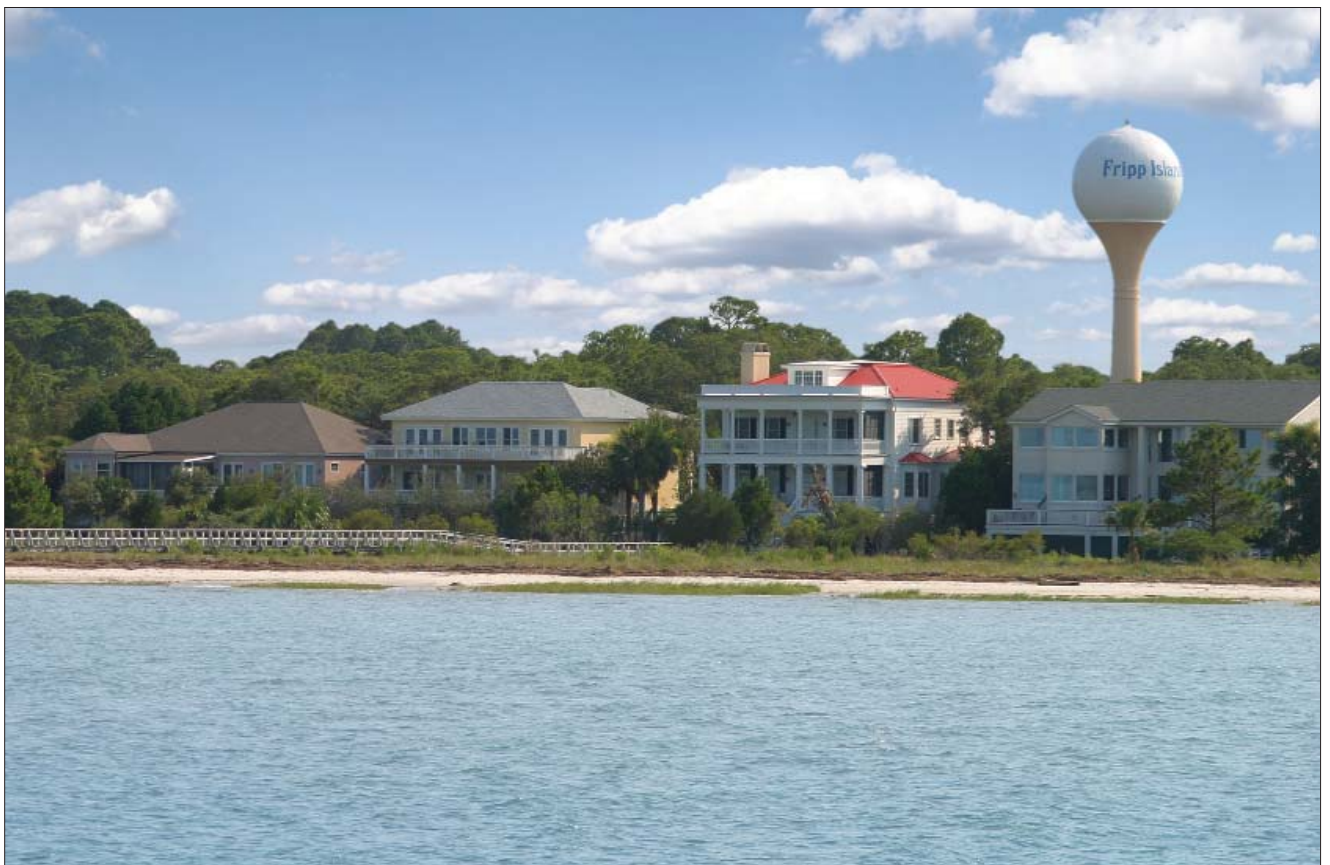
Vacuum sewer technology is a cost-effective solution for communities with flat topography, sandy soil, and a high water table, like Fripp Island, SC.
