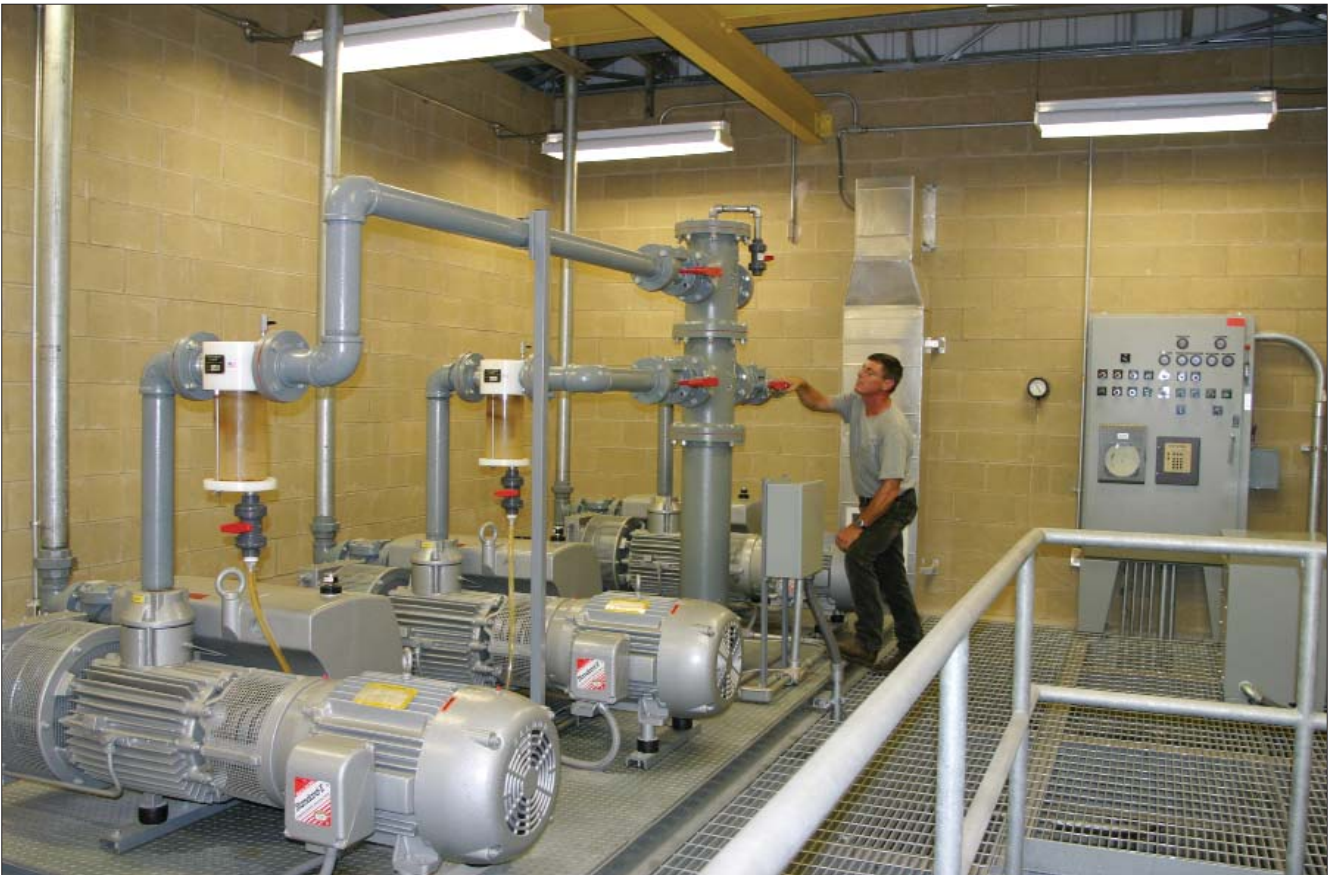
Vacuum sewer stations provide a clean, odor-free working environment, and because vacuum sewers are a closed system, workmen never come in contact with raw sewage.
