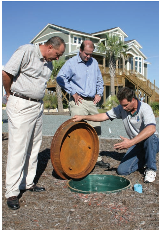
Frank Bland, AIRVAC regional manager (left), and Bart Sanders, AIRVAC field representative (right), explain how a vacuum valve pit works to Steve Wheeler, Holden Beach town manager (center).
