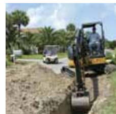
Small equipment reduces neighborhood disruption.
