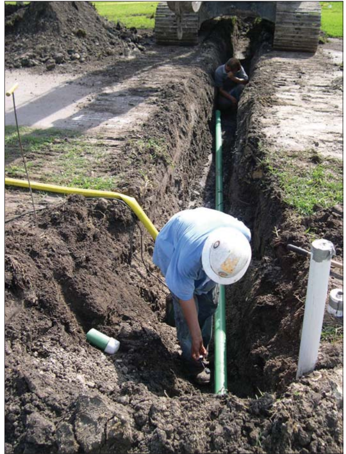
Vacuum sewer service lateral installation is simplified because lines are shallow and can easily be diverted over or under buried obstructions.
