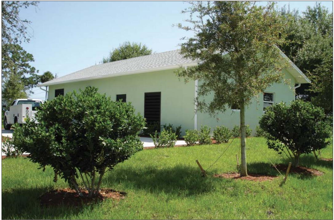
Single vacuum station, which services all of Rockridge's 400-plus houses, features an attractive stucco exterior that matches local architecture.
