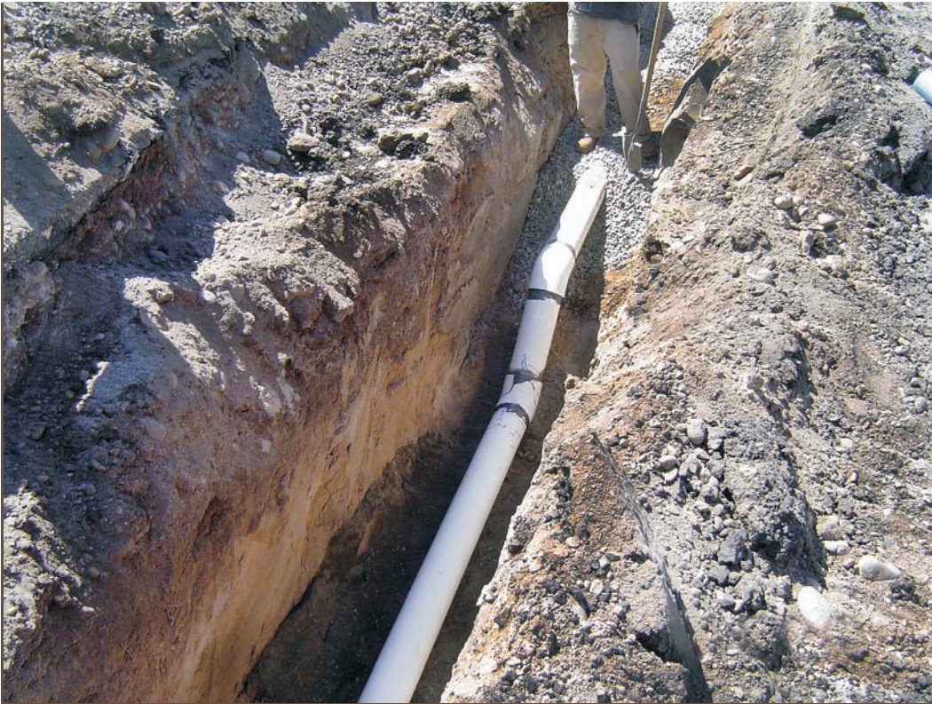
AIRVAC vacuum mains have a "sawtooth" profile that helps maintain negative pressure within the pipeline and allows for shallow burial depths, typically 4-6 feet deep.
