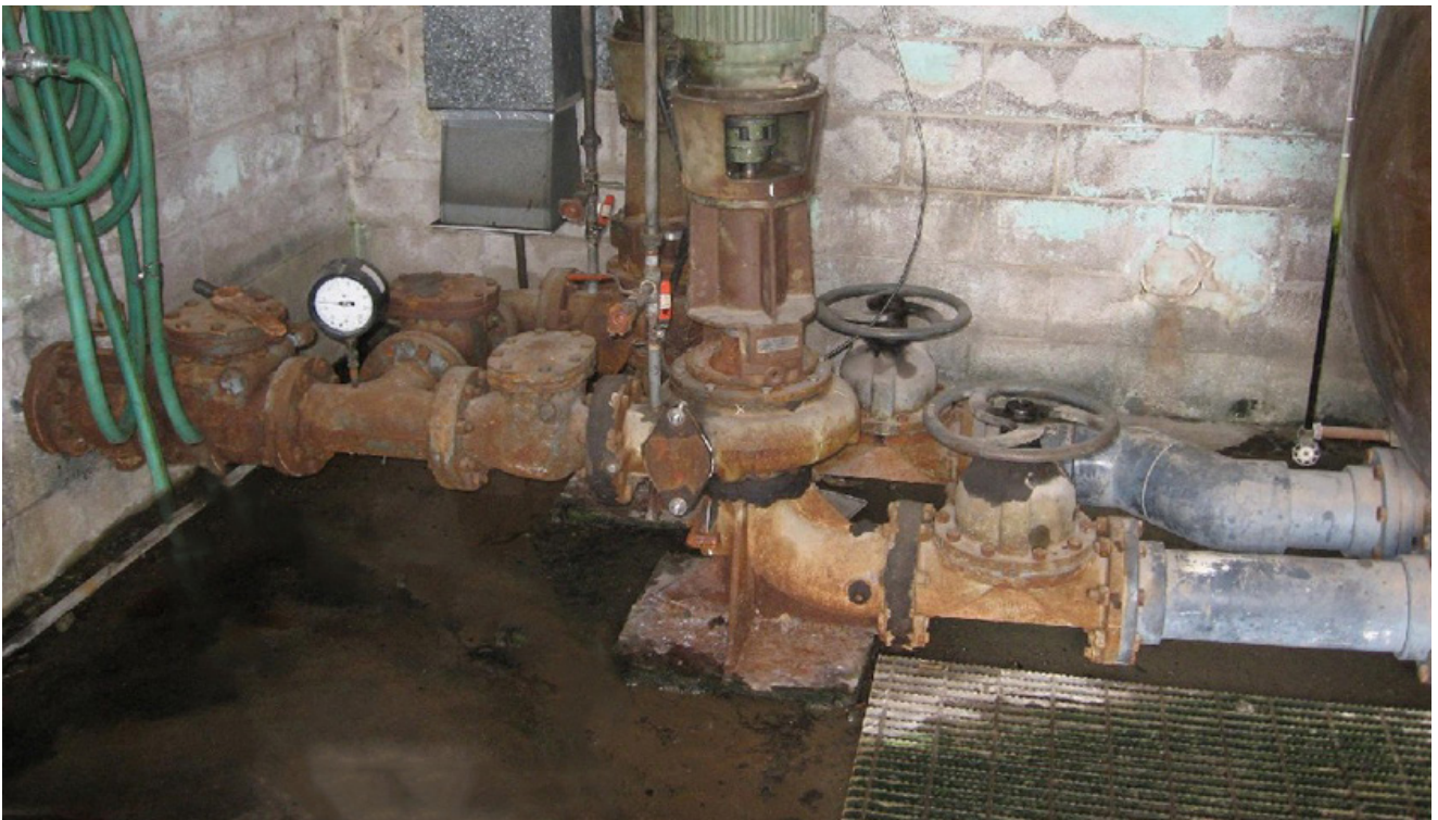
These sewage pumps were originally installed in 1978 and continue to operate.
