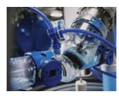
The Airvac vacuum valve opens when 10 gallons of sewage collects in the sump and then differential pressure propels the contents into the vacuum main.
