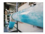
Wastewater travels at 15 to 18 fps in a vacuum main, which is laid in a sawtooth fashion to ensure adequate vacuum levels at the end of each line.
