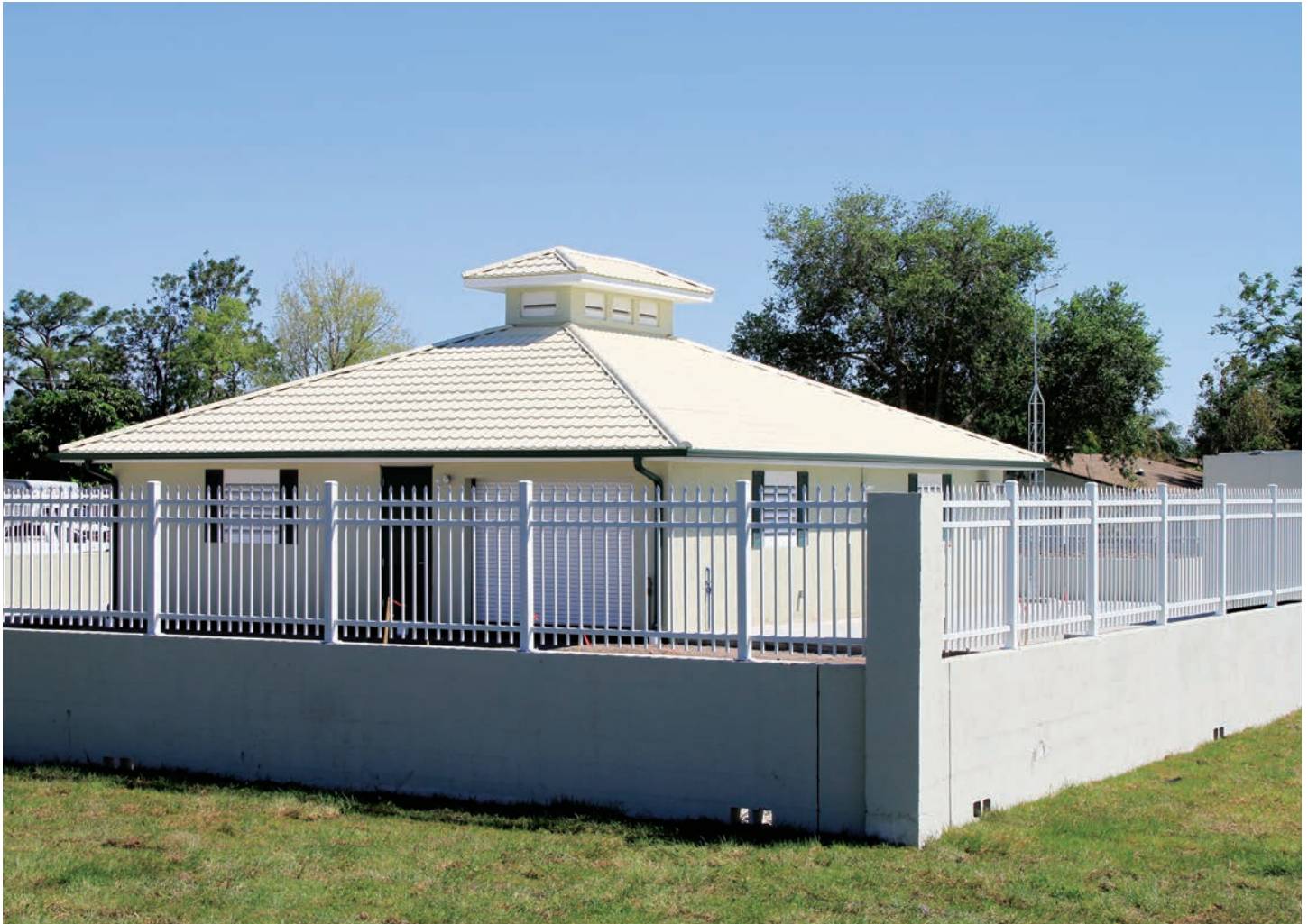
Vacuum stations cover a relatively small footprint, are odor free and can be designed to blend into the neighborhood.
