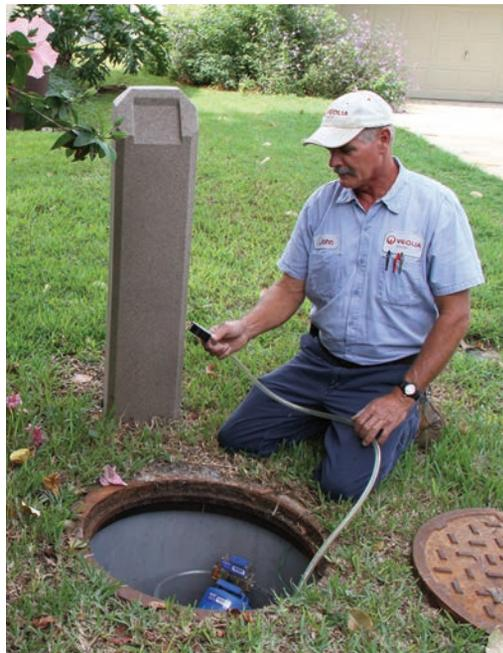
Veolia Field Supervisor John Morris checks the vacuum level in Crystal River's AIRVAC sewer system as part of a scheduled maintenance program.
