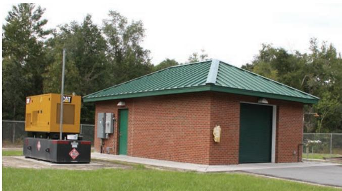
This vacuum station is equipped with a backup generator in the event of power loss due to hurricanes, tropical storms or severe thunderstorms.
