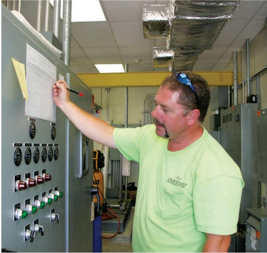
**Monitoring systems in the central vacuum station can help locate a malfunctioning valve. Repairs to stuck valves usually take only a few minutes.**
