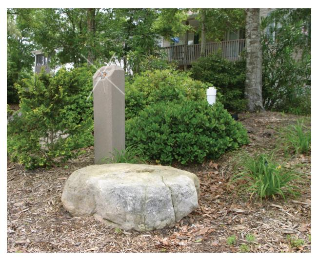
The solar light monitor is easily visible from a long distance, avoiding the need for operators to physically check every vacuum valve in the system.
